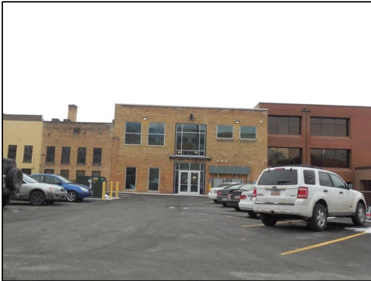
Implement Building 2314 South Washington Boulevard Ogden, Utah
