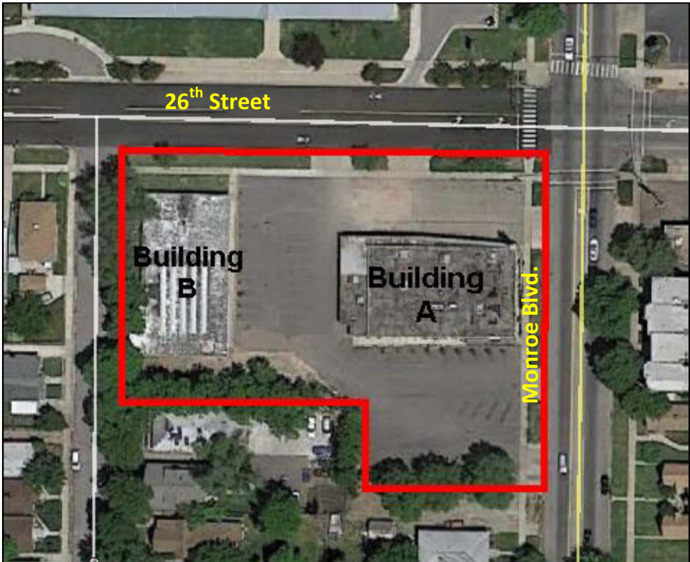
Property Aerial View
