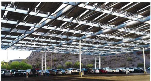
(UofU canopies would have lower maximum height than these examples, but still provide minimum 14'-0" clearance to enable all freight deliveries, future paving maintenance, and snow removal by existing campus fleet)
