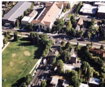
Aerial view of the intersection of 700 North and 800 East. A major activity node should be established to increase pedestrian activity and entrance awareness.
