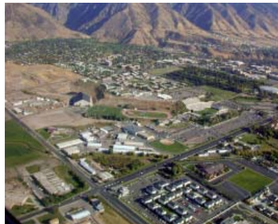
Aerial view of the motor pool and storage area (lower center). This area will transition to house major services such as purchasing, personnel, police, parking, facilities, printing, and photography.
