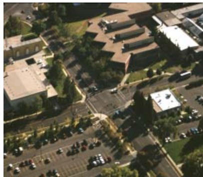
Aerial view of the intersection of 700 North and 1200 East where a major activity node should be created.
